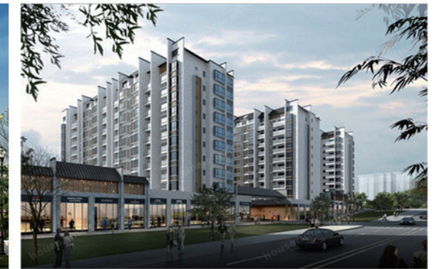
福建龙岩万星豪庭 Project Huating Hotel in Fujian
